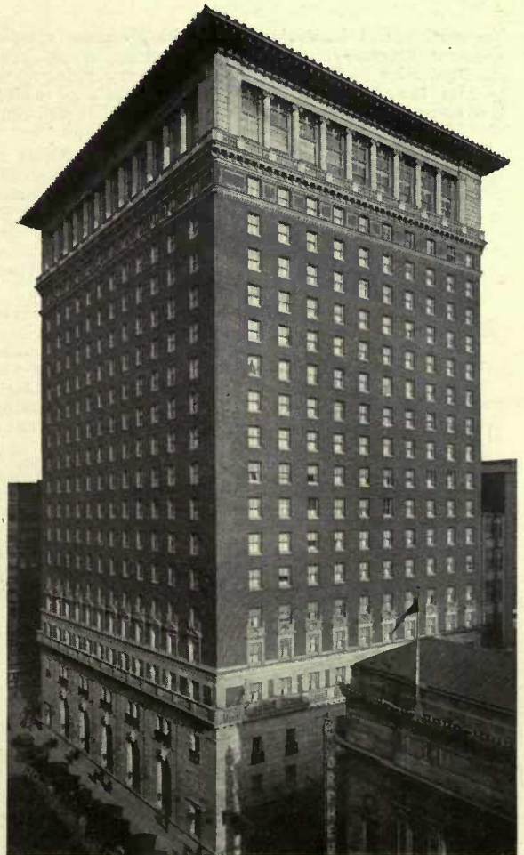
Statler Hotel, St. Louis, Mo. Mauran, Russell & Crowell and Geo. B. Post & Sons, Associated Architects Construction work below grade waterproofed with Truscon Water- proofing Paste, Concentrated .
